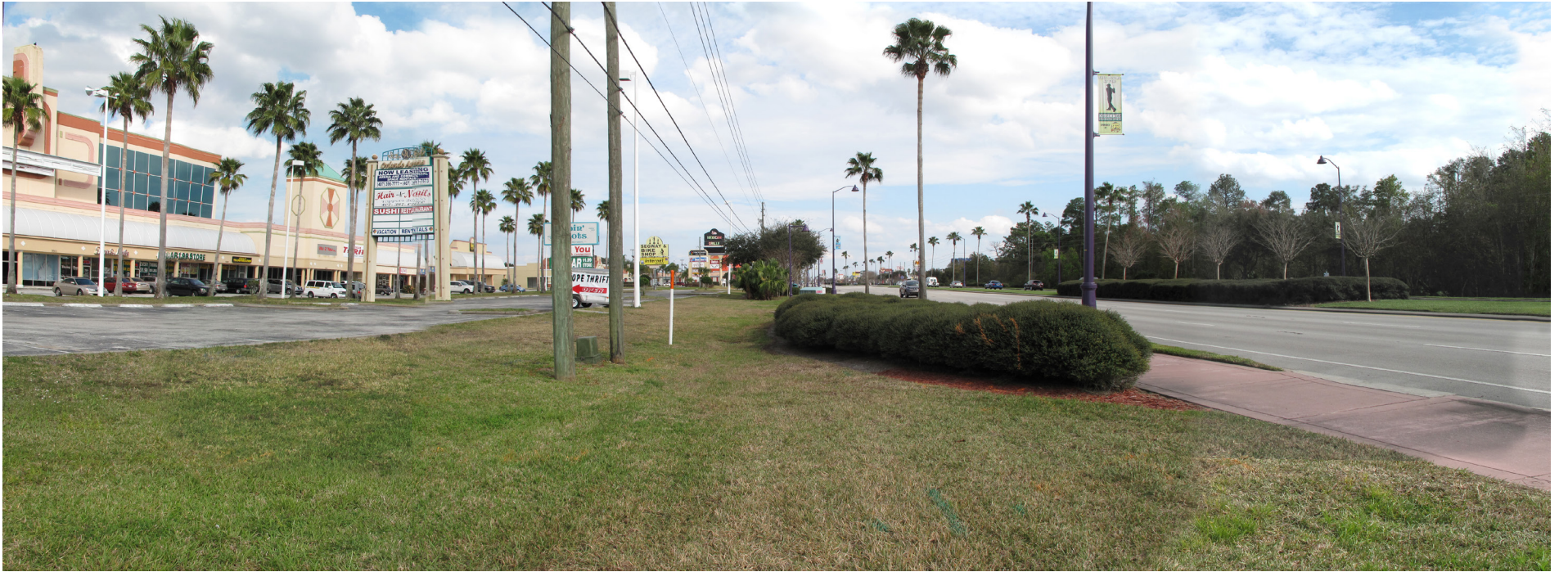
Typical Existing Condition
